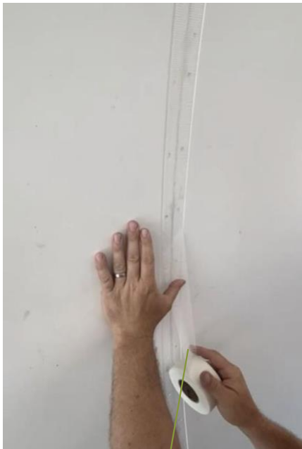
FIBERGLASS MESH ADHESIVE TAPE OR TAPE
