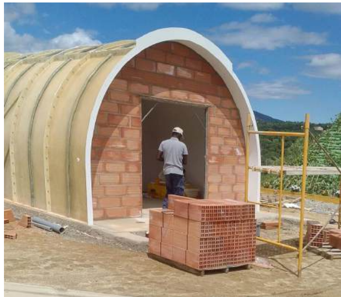
Figure 2. Construction of a W.S.
